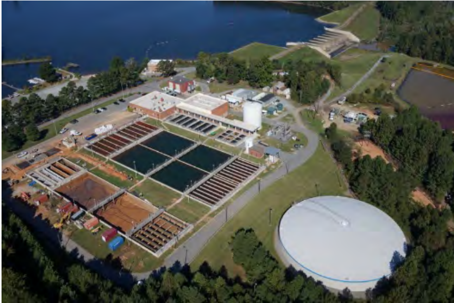
Lake Townsend Water Treatment Plant
